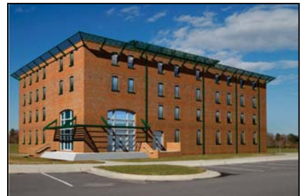
Picture 2: Center for Business Development
